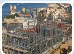
system, which is fixed as a rapid dry infill between the main structural frame members. The system acts as a carrier for external cladding, internal wall make-up and insulation. ASF is designed to suit the loading, deflection and dimension requirements of each project. The cold rolled galvanised framing consists of
